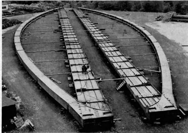
Fig. 15: Assemblage of the main girders in the steel construction workshop
