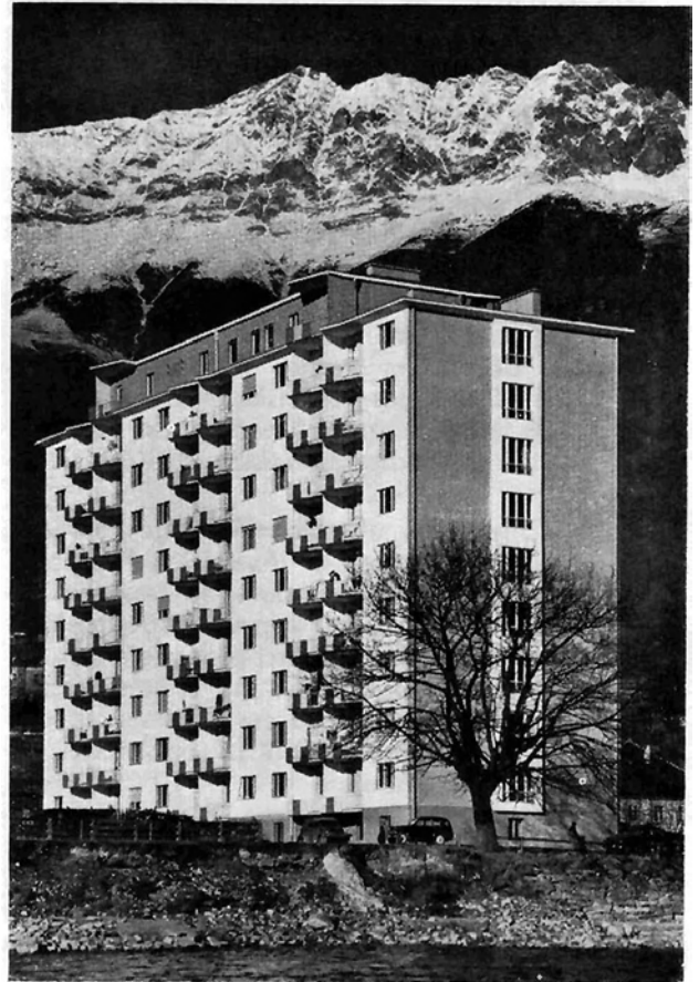
Fig. 9: Multi storey building, University Bridge, Innsbruck, in light skeleton construction. For this design only 2/3 of the normal steel quantity were required
