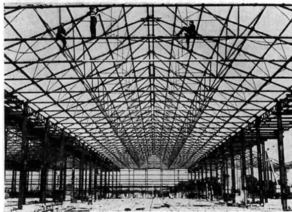
Fig. 5: Diffusion building at Capenhurst — principal trusses of tubular construction
