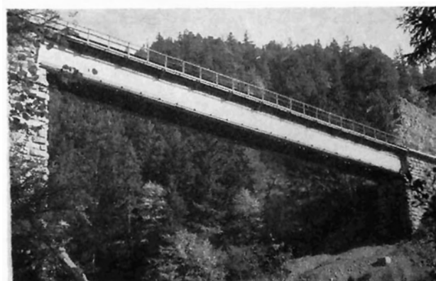
Fig. 7a: Disassembly of the old bridge
