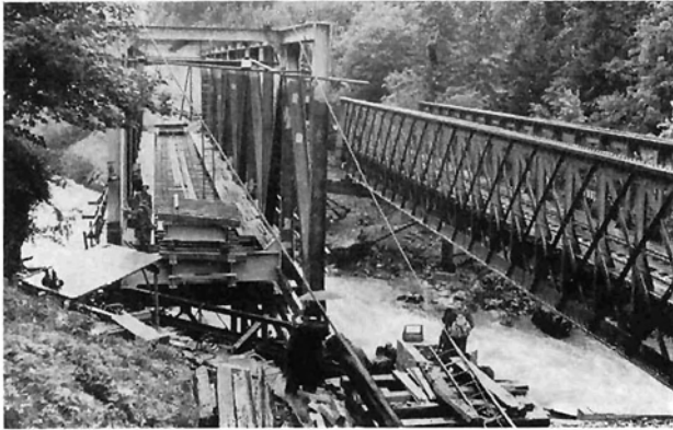
Fig. 8: Kummer-Bridge; Erection
