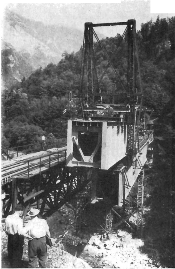
Fig. 4c: New bridge, erection
