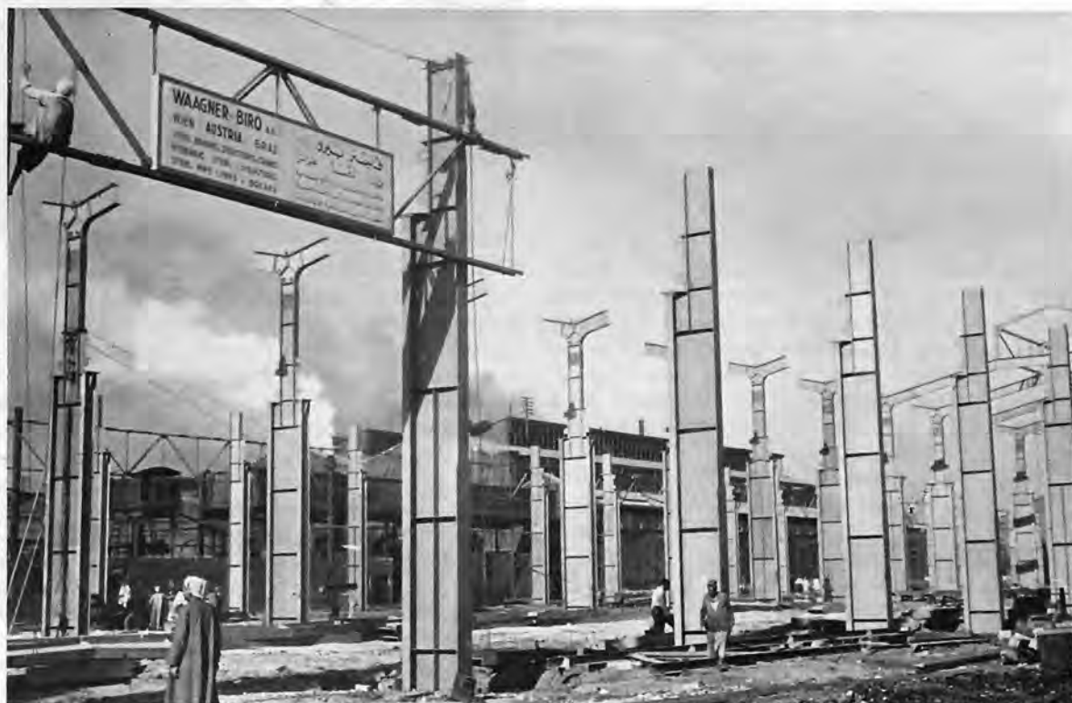
Fig. 1: Working state of the "Diesel"-Locomotive Shed with erected main supports
