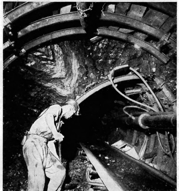
Fig. 10: Pipe rollers as supporting parts for the rubber belts of conveyor plants
