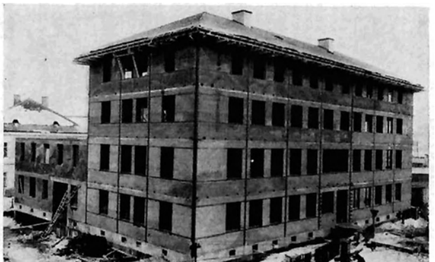
Fig. 4: Crude construction finished and roofed
