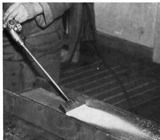
Fig. 3: Derusting of a channel iron
