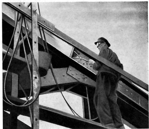
Fig. 3: Flame cleaning of a bridge, width of burner 300 mm
