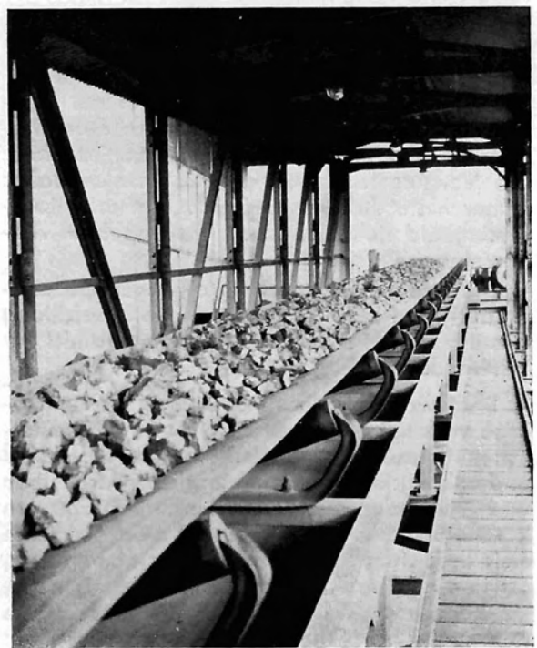
Fig. 7: Belt conveyor bridge for transportation of wood chips, paper factory Gratkorn of Messrs. Leykam-Josefsthal AG.
