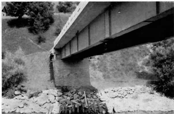
Fig. 12: Compound girder bridge with prefabricated concrete slabs
