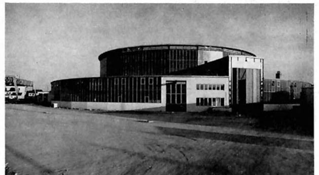
Fig. 41: Total view of a round-shaped hall with suspension cone roof at Gleisdorf, Styria
