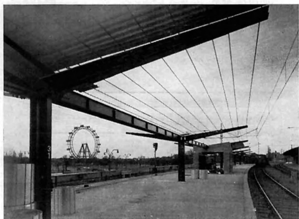
Fig. 38: Prestressed steel wire roof, acc. Maculan, for a local railway station in Vienna
