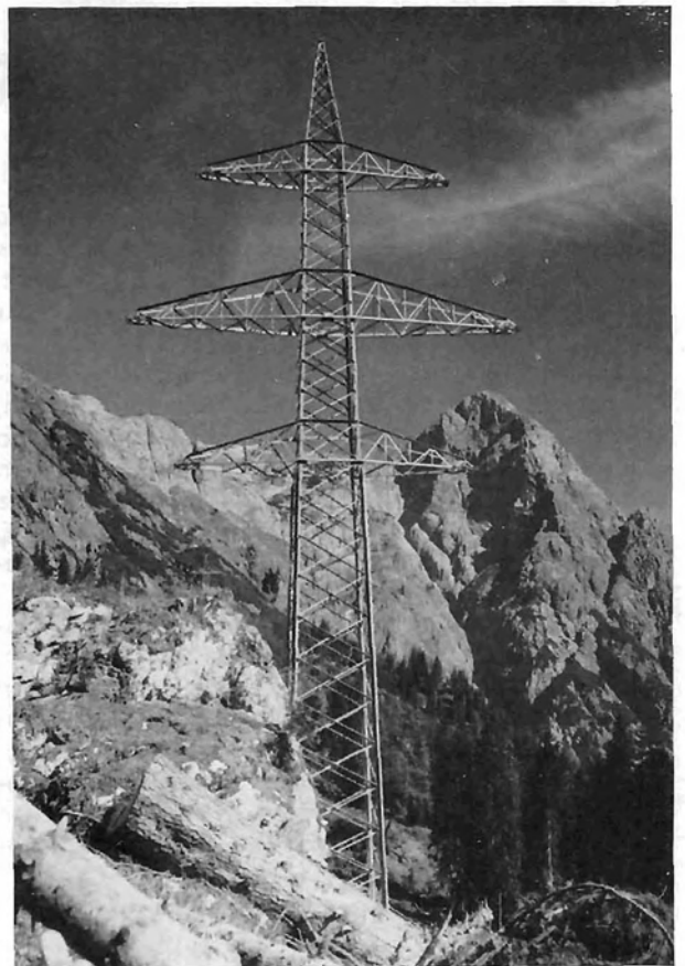
Fig. 17: 220 kV Tension tower in high mountain region
