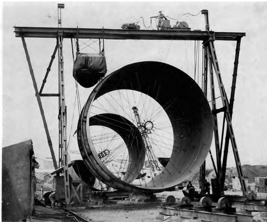
Manufacture of pipes (8 m diam.) on Seyhan site, Turkey.
