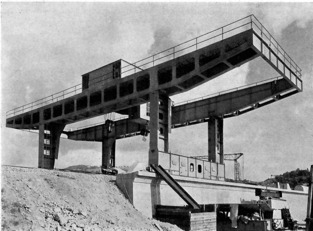
Crane for the hydro electric power plant Rosenau
