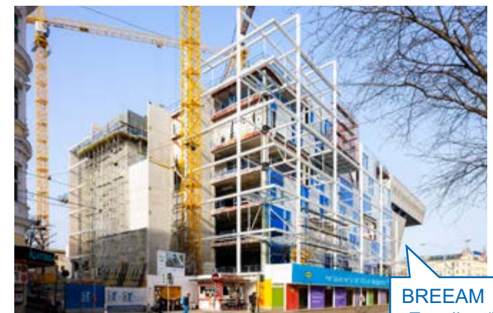
Baufortschritt in Natura
