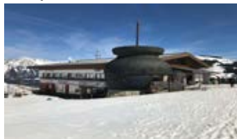
ALTE STATION (ABBRUCH)
