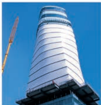
EUROPEAN STEEL DESIGN AWARD 2005 – AIR TRAFFIC CONTROL TOWER – AIRPORT VIENNA
