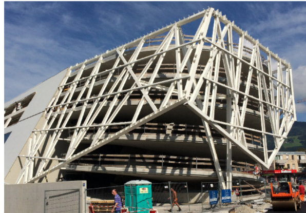
STAKO Fassade Süd West Wendelrampe: Primary + secondary
