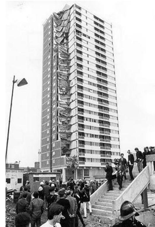
**Ronan Point** was a 22-story tower block in Newham, east London, which suffered a partial collapse when a gas explosion demolished a load bearing wall, causing the collapse of one entire corner of the building. Four people were killed in the incident, and seventeen were injured.
